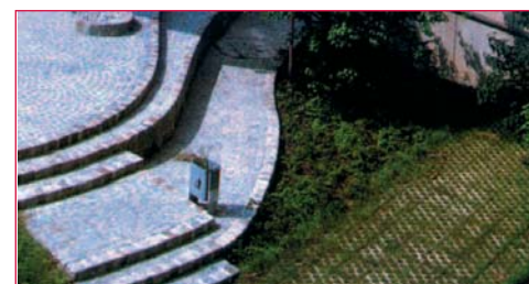
Porous paving as a garden pathway
